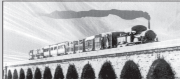
Train passing through India's first creek bridge near Thane - 1854
